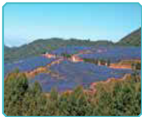
Yunnan Menghai Solar Power Plant
