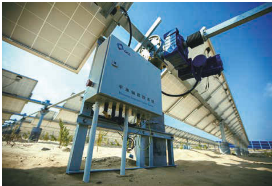
Horizontal single axis smart tracking system
