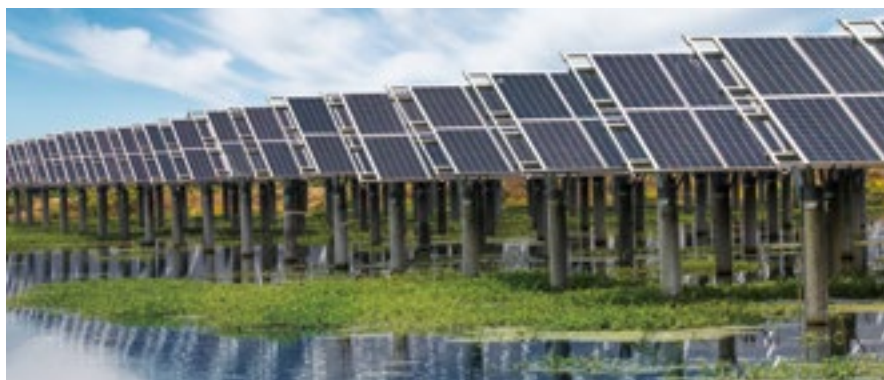
▲ Fishery complementary solar power plants in Tianchang, Anhui Province
