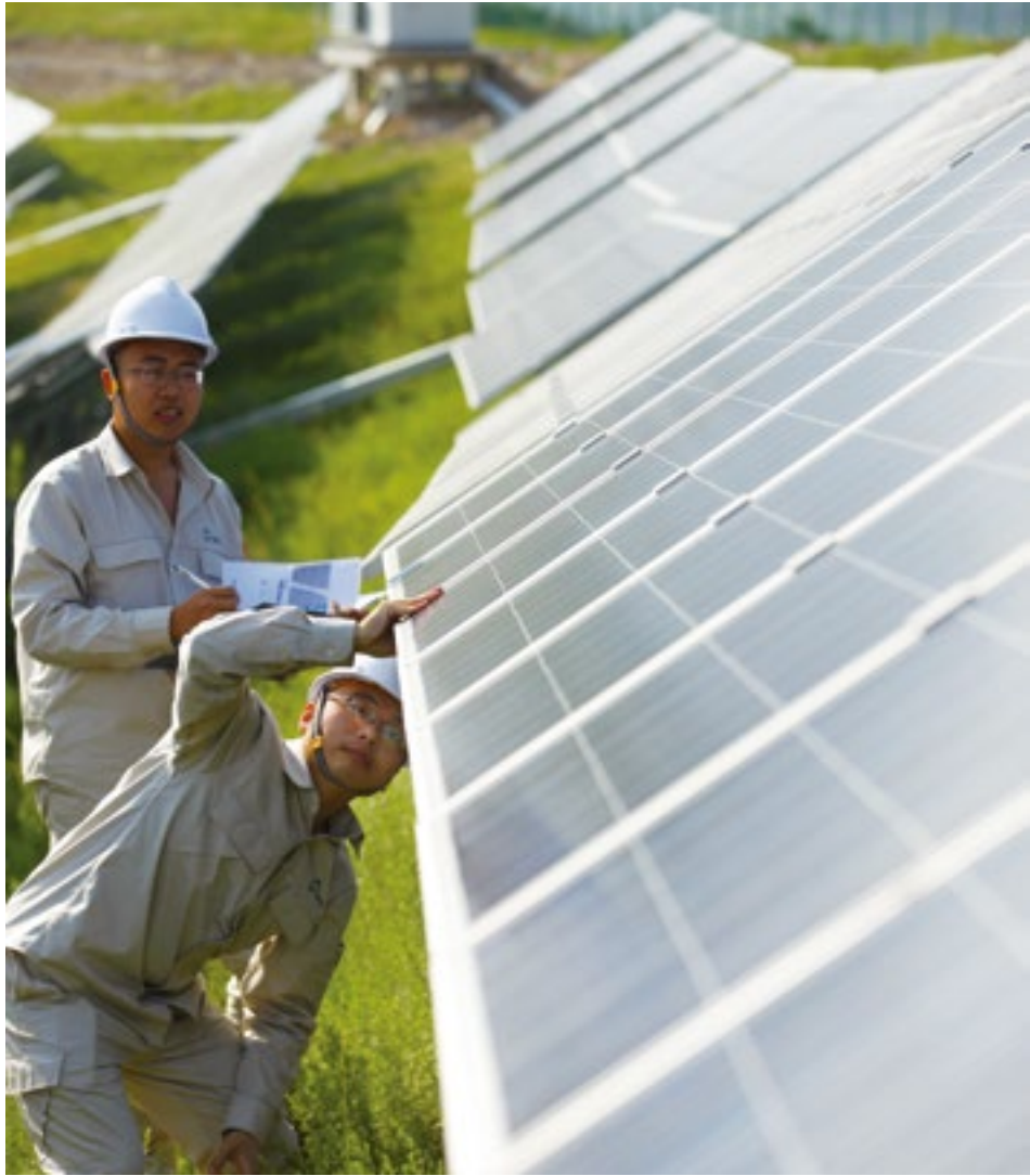
▲ Repairing photovoltaic modules in Licheng, Shanxi Province
