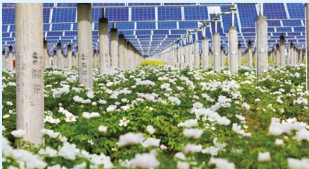
▲ The Solar Energy + Peony power station with a capacity of 40MW in Suzhou.
